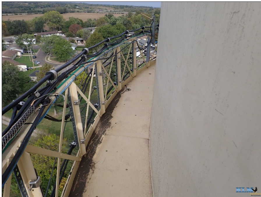
Photo No. 34 Balcony and handrail
