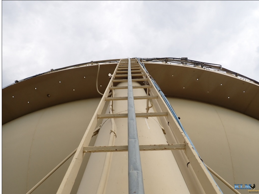
Photo No. 37 Column ladder and underside of balcony
