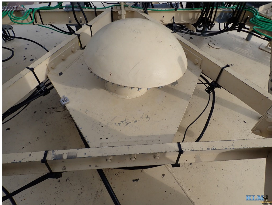
Photo No. 22 Finial vent
