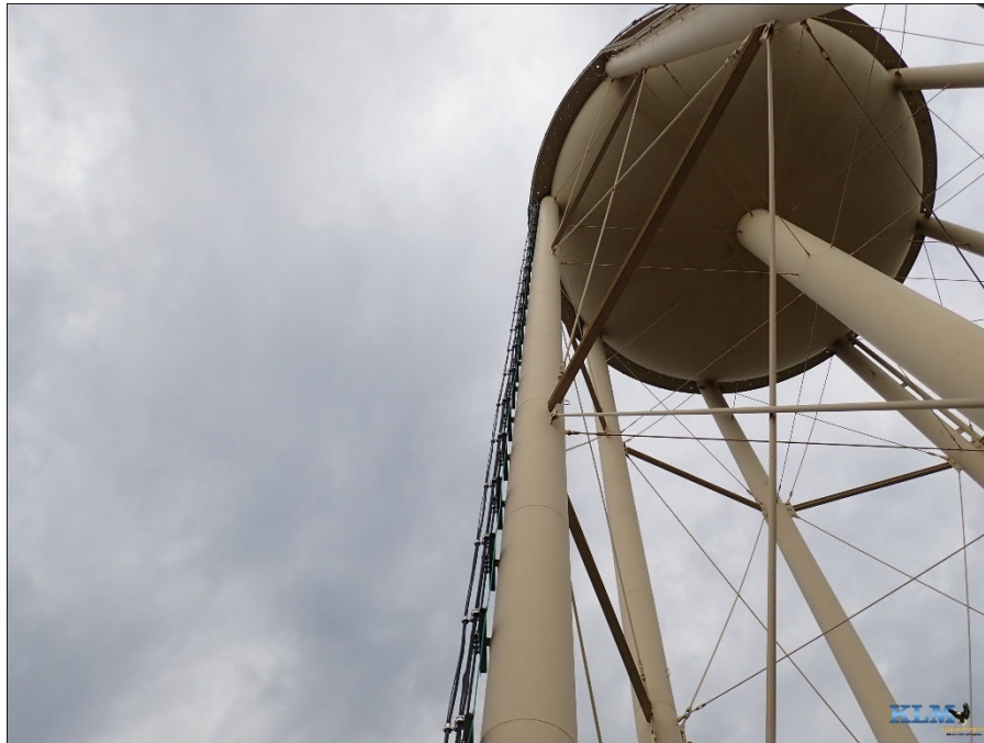
Photo No. 40 Antenna cables and mounts on column
