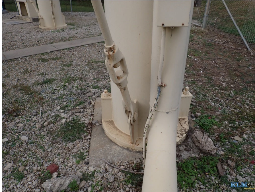
Photo No. 49 Column, overflow pipe, and footing
