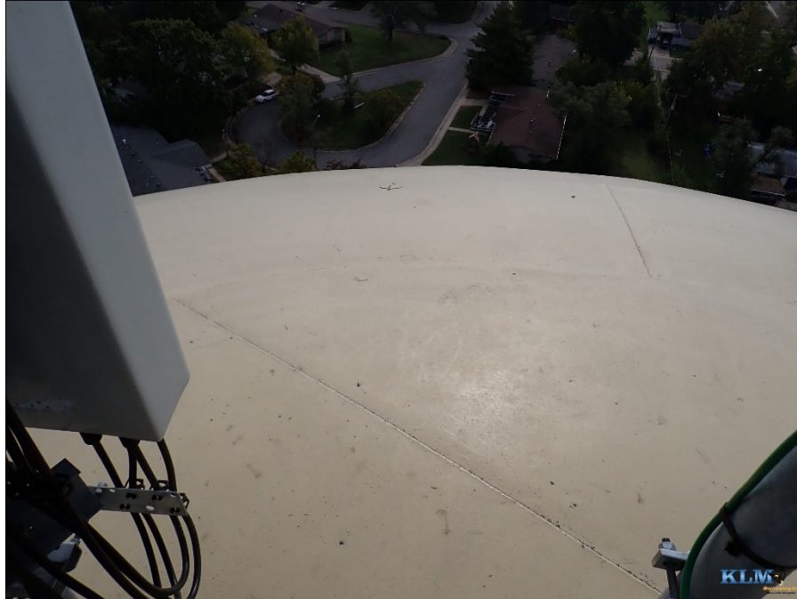
Photo No. 27 Roof coating conditions
