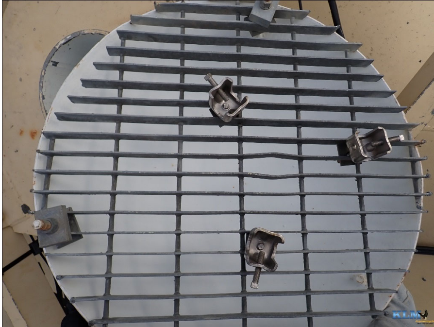
Photo No. 23 Underside of vent cover
