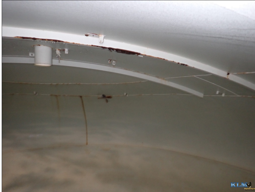
Photo No. 3 Roof coating conditions
