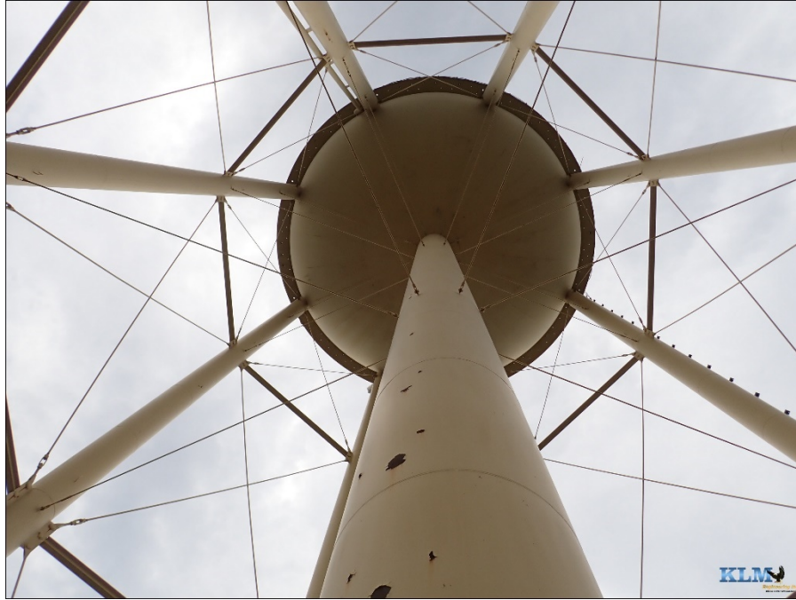
Photo No. 39 View of bowl, wet riser, and columns
