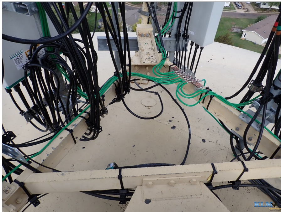
Photo No. 18 Antenna mount assembly on roof
