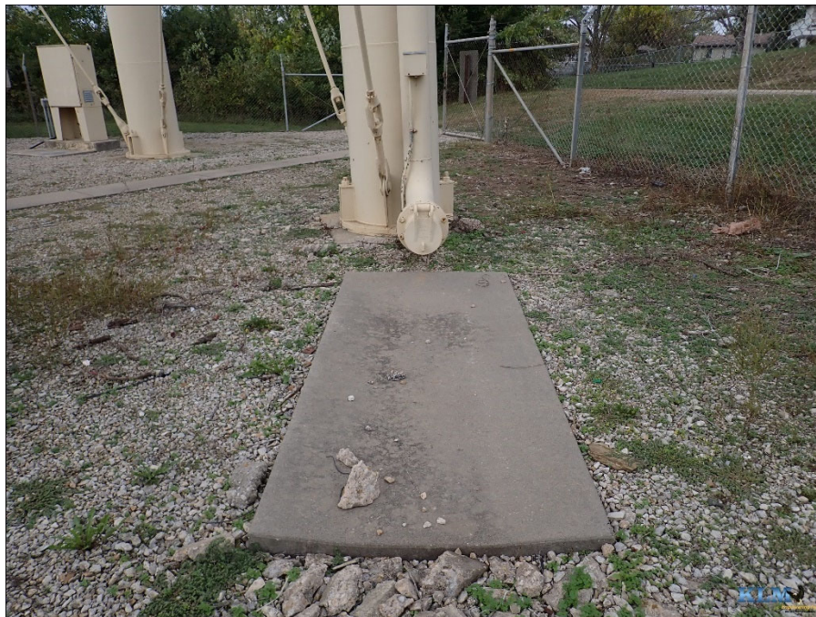
Photo No. 50 Overflow pipe outlet and splash pad
