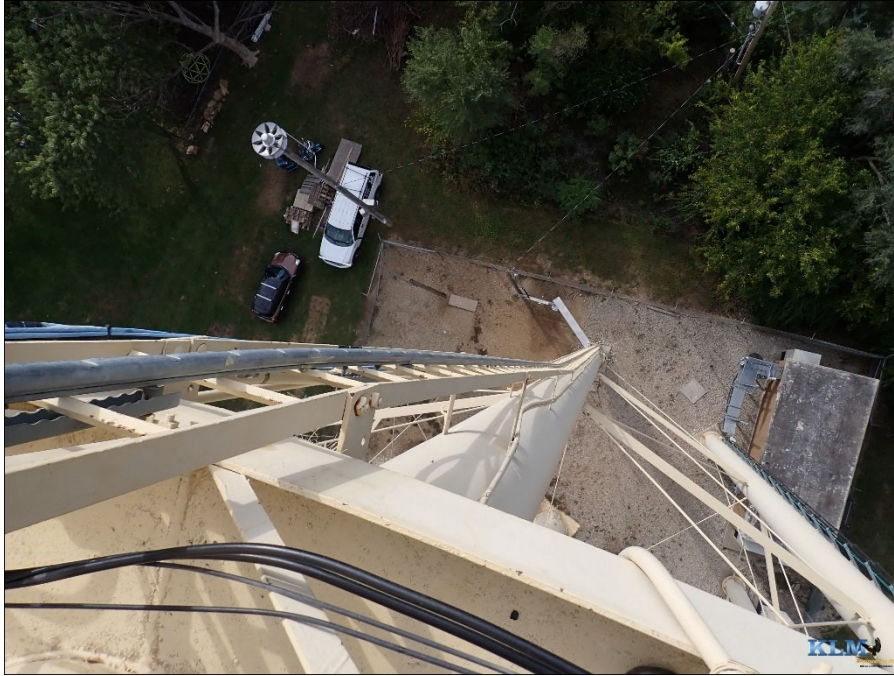
Photo No. 35 Column ladder
