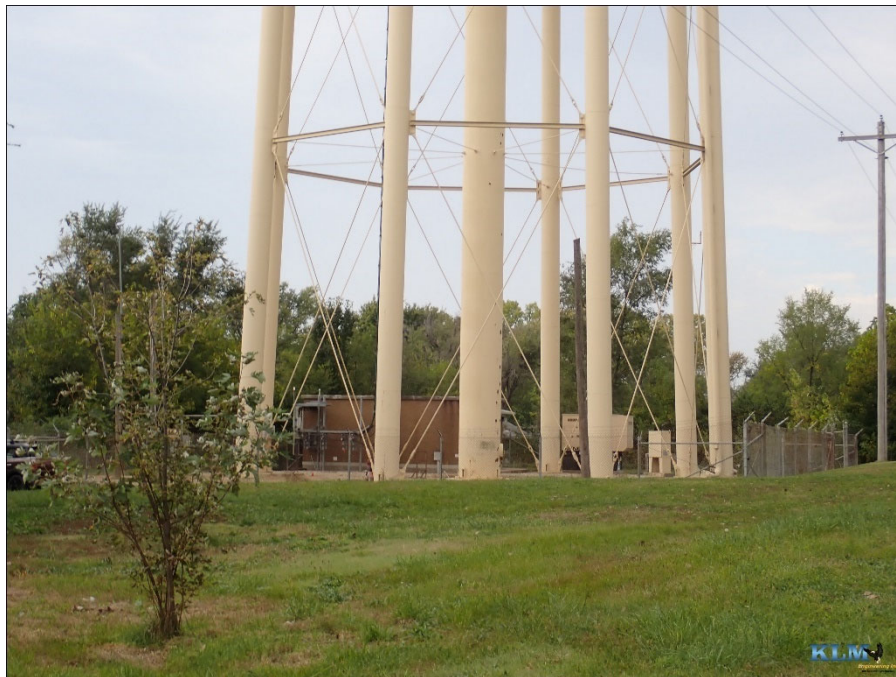
Photo No. 52 Site conditions
