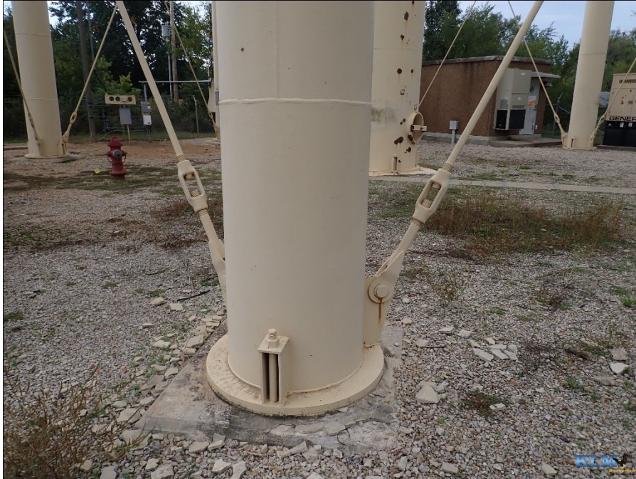
Photo No. 47 Column and footing
