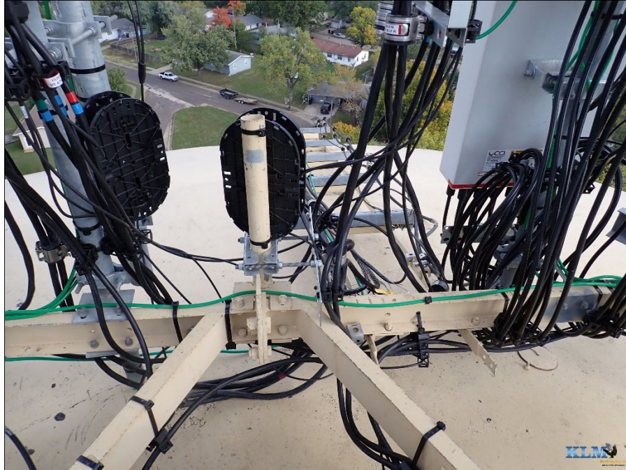
Photo No. 19 Antenna mount assembly on roof
