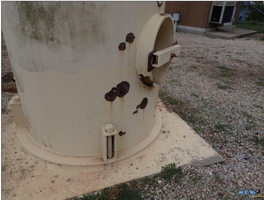
Photo No. 44 Bottom of wet riser Manway visible
