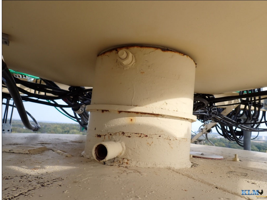
Photo No. 25 Underside of vent platform
