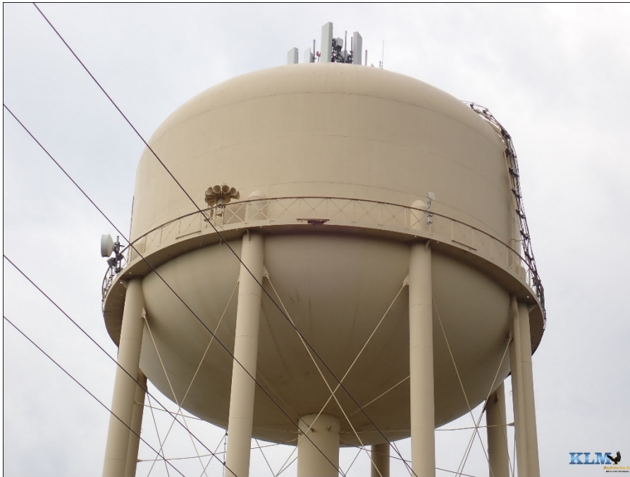
Photo No. 36 View of water compartment
