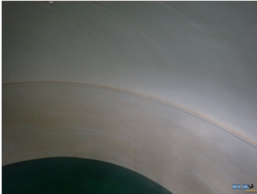
Photo No. 7 View of upper torus and shell Stiffener ring visible
