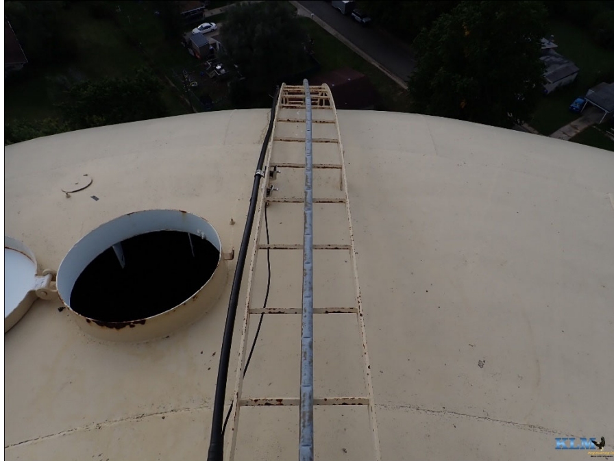
Photo No. 29 Wet access manway and roof ladder
