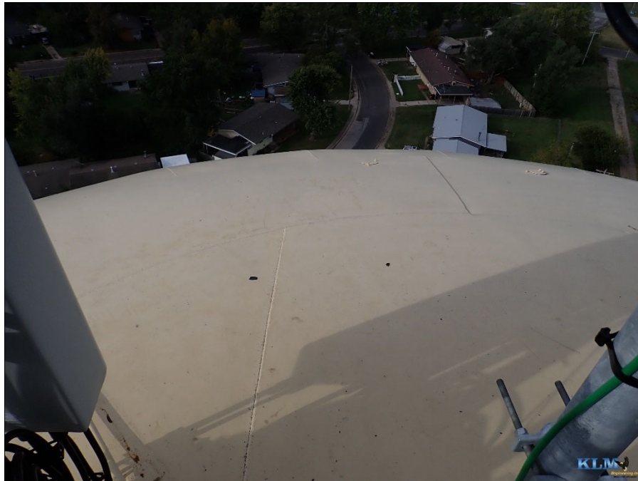
Photo No. 28 Roof coating conditions
