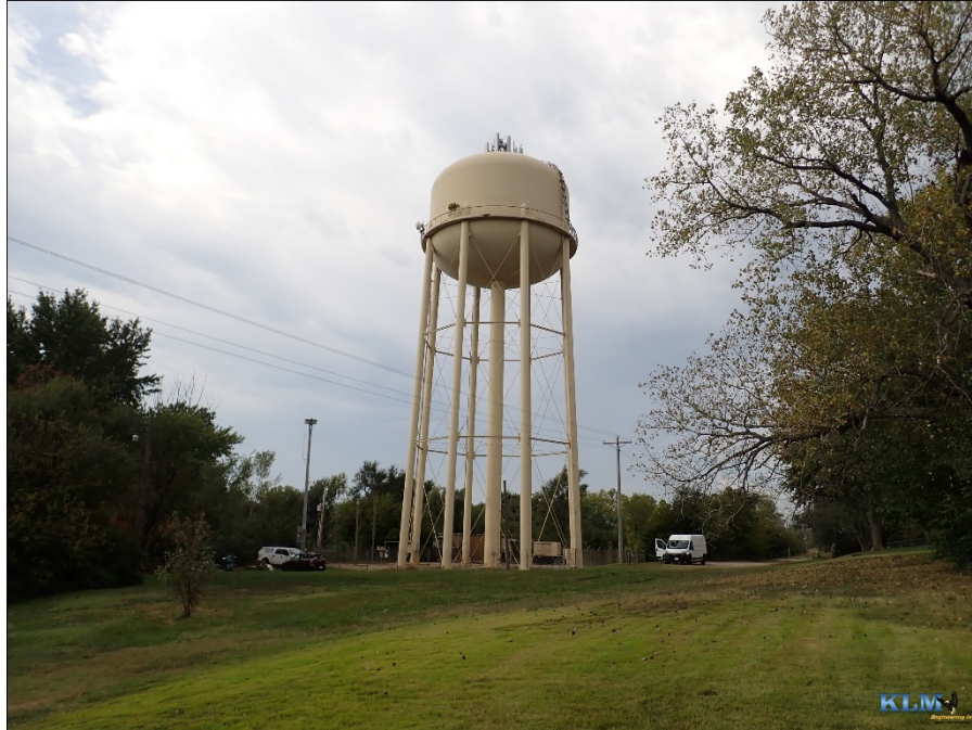
Photo No. 1 Overall view of the tower
