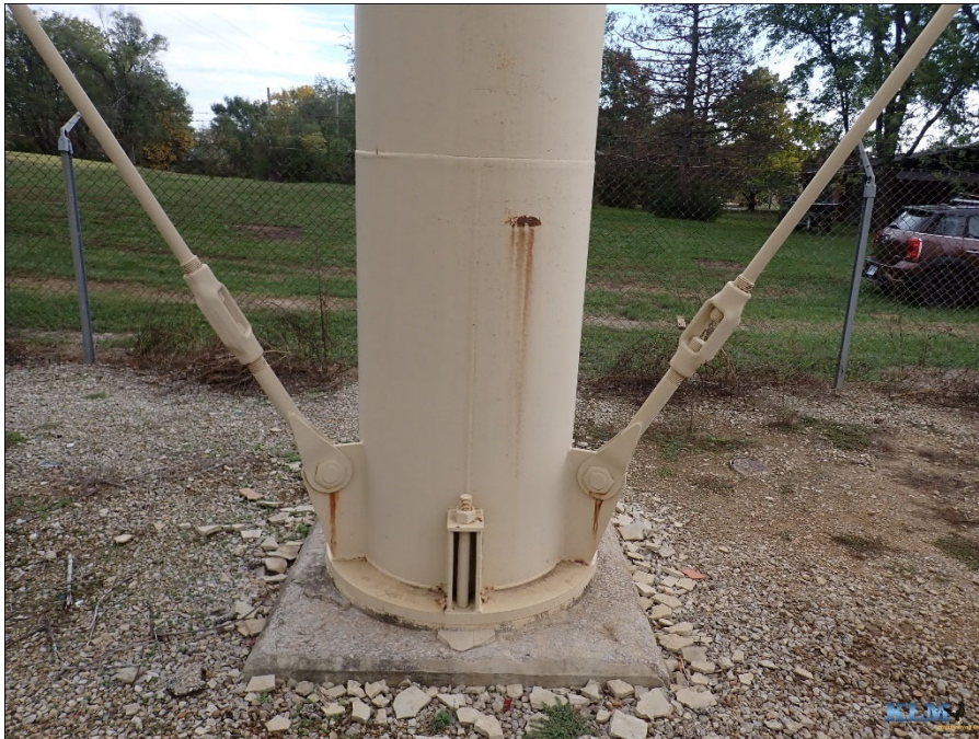
Photo No. 46 Column and footing
