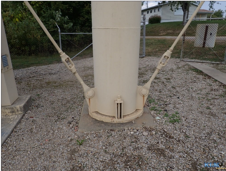
Photo No. 48 Column and footing
