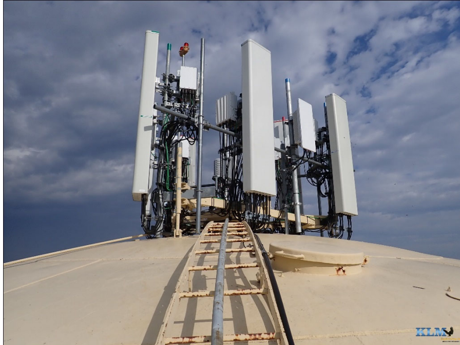
Photo No. 17 View of roof
