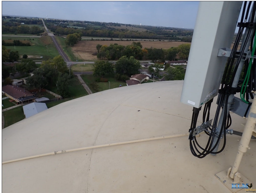
Photo No. 30 View of roof and upper torus Conduit visible
