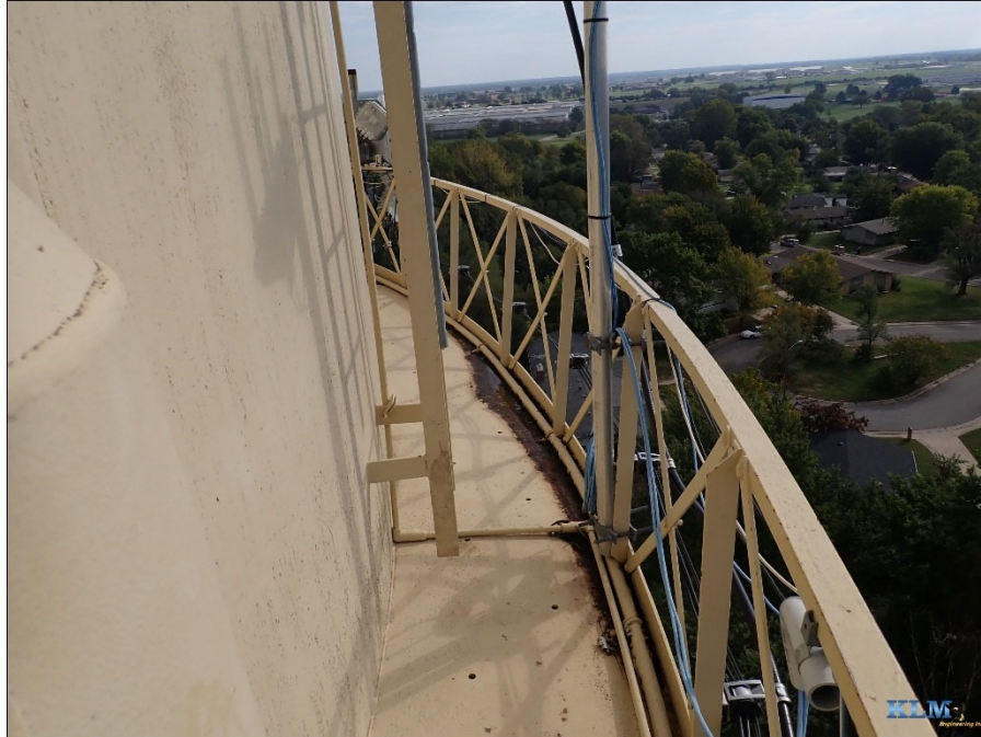
Photo No. 33 Balcony and handrail
