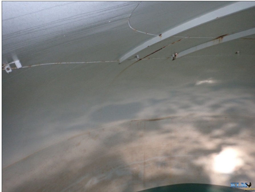
Photo No. 4 Roof coating conditions
