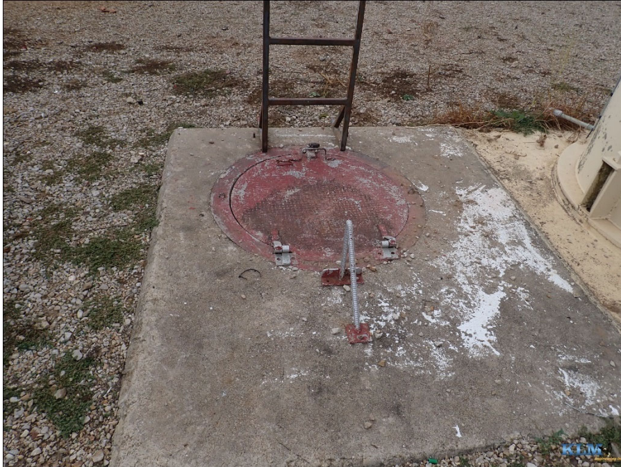
Photo No. 45 Valve pit access
