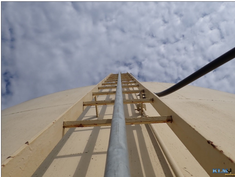
Photo No. 32 Shell ladder
